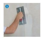
Lay the reinforcement strips in the filler 2...
