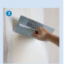
VARIO joint filler or ProMix Plus should also be used for subsequent filling. Do not apply further filler until the preliminary layer is dry 4.
