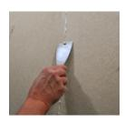
For a perfect appearance, screw heads and surface defects should be filled and the adhesive joint covered with a layer of VARIO joint filler or ProMix Finish ready filler once it has fully hardened.
