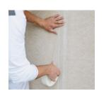
**Preliminary filling:** Apply VARIO joint filler with a smoothing trowel and level to the height of the edge.
