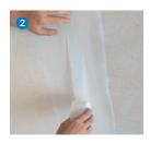
... and then smooth the filler over without applying further material 3.
