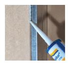
Press the next board against the first leaving a joint gap of max. 1 mm. The joint adhesive must fill the entire joint when the boards are pressed together.
