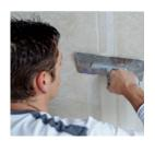
**Subsequent filling work:** Further filler may only be applied once the previous layer has fully hardened. Use the same material as for preliminary filling or Rigips ready filler (ProMix Finish).
