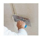
Subsequent filling work: Further filler may only be applied once the previous layer has fully hardened. Use the same material as for preliminary filling or Rigips ready filler (ProMix Finish).
