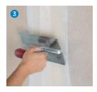
Use VARIO joint filler or alternatively ProMix Finish for subsequent filling. Do not apply further filler until the preliminary layer is dry 4.
