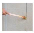
**Preliminary filling:** Apply VARIO joint filler with a scraper or smoothing trowel at right angles to the joint and level with the surface. Fill holes / defects and cover screw heads with joint filler.
